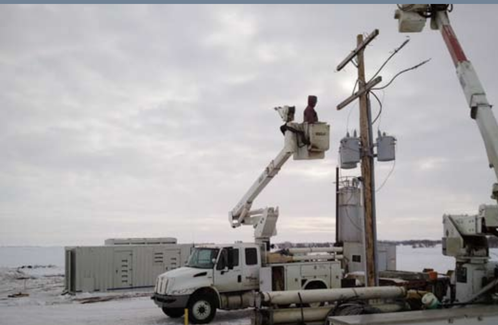
Tapping into the line as it goes out to flare, gas is captured and run it to the generator, which then provides power that can be returned into the power grid or used on-site. Photo provided by Blaise Energy.
