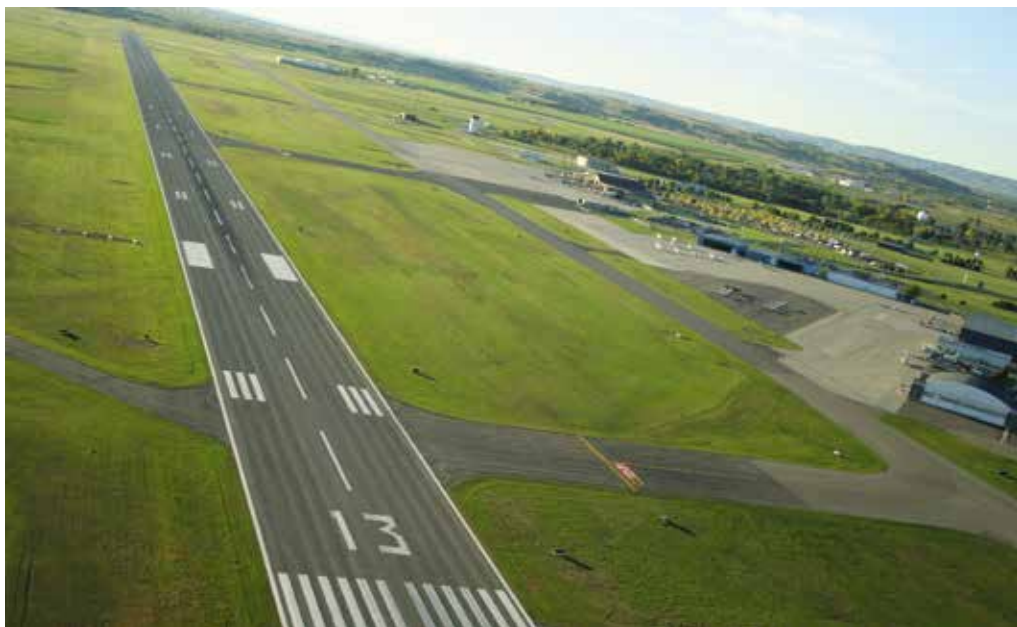
An aerial shot of Bismarck Airport. KLJ was recently selected to serve as Bismarck Airport's engineering consultant for the next five years. KLJ has served as their airport consultant since 2009, leading multiple capital improvement projects in collaboration with airport staff.
