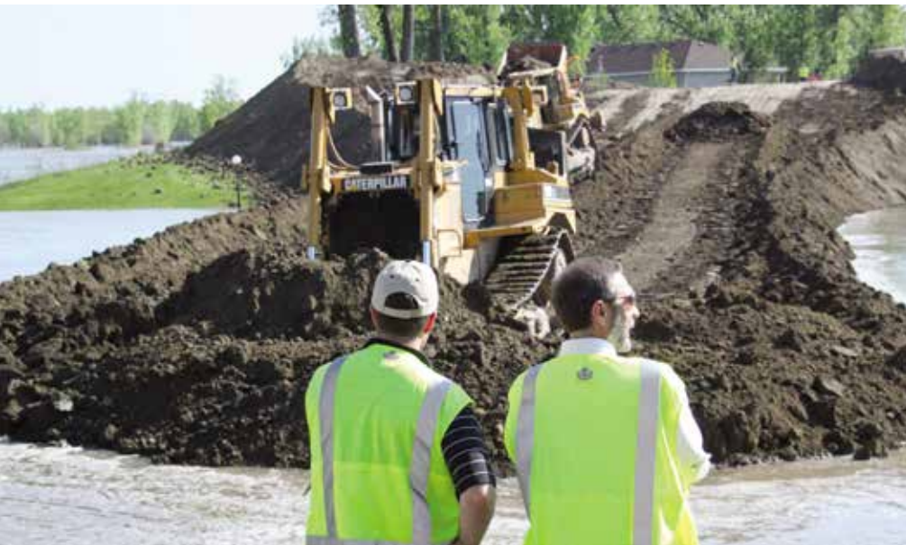
KLJ proposed an emergency plan to construct clay plugs in three of Mandan's marina inlets to protect 250 residences and $70 million of public infrastructure during flood events in 2011. Above, Niles Hushka, KLJ's CEO, oversees construction of the clay plugs.
