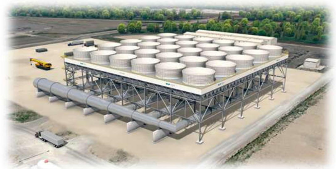
Air Cooled Condenser
